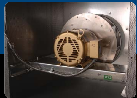
Smaller fans running at higher speeds reduce sound levels and attenuation costs. They also promote easier maintenance.
