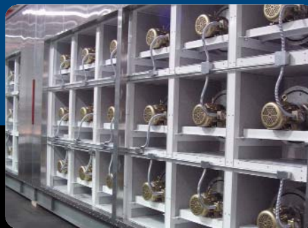
Smaller fans running at higher speeds reduce sound levels and attenuation costs. They also promote easier maintenance.
