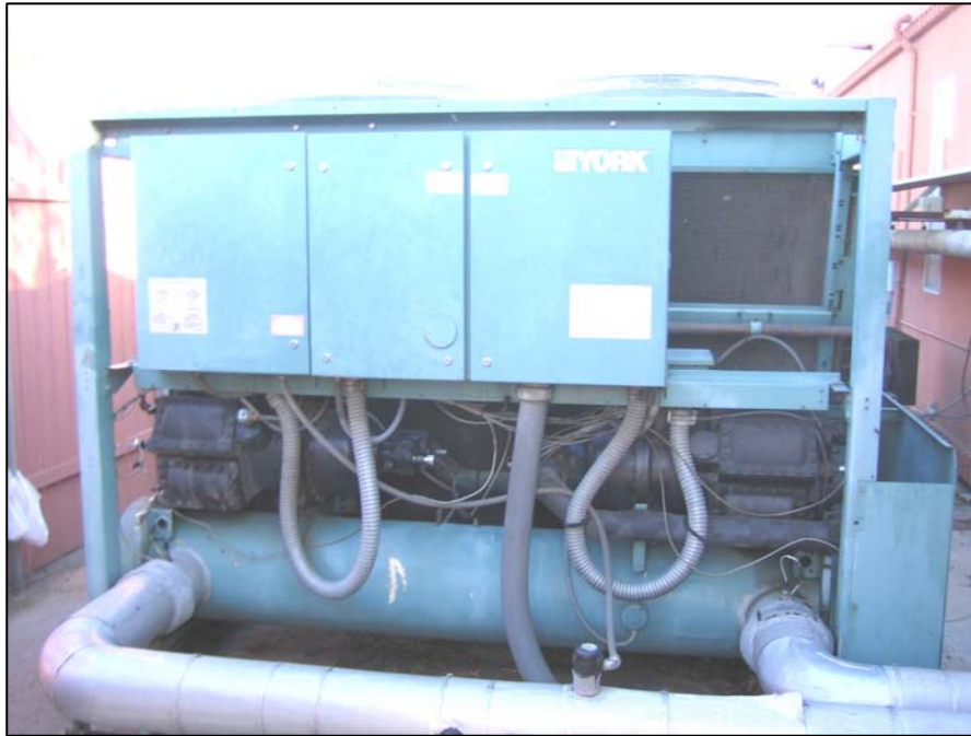
Figure 1: York air-cooled chiller (model YCA288HE3)
