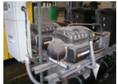
Thermal Care chiller package features oil-free Turbocor compressors.
